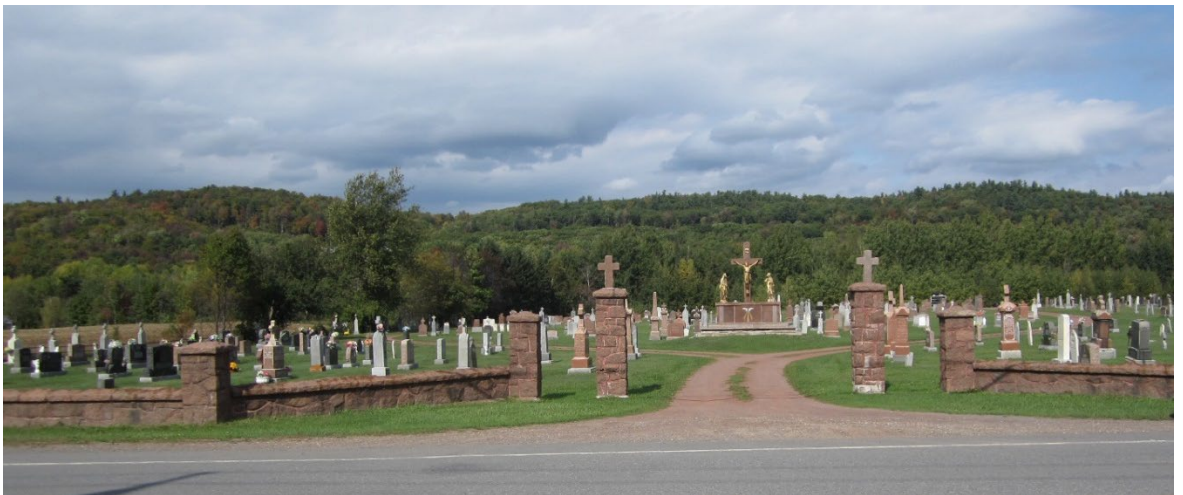
ORNAMENTAL FENCE ALONG THE FRONT OF CIMETIÈRE CALUMET-GRENVILLE, IN THE FORM OF A LOW WALL AND COLUMNS IN PINK GRANITE (GSLR-29).
