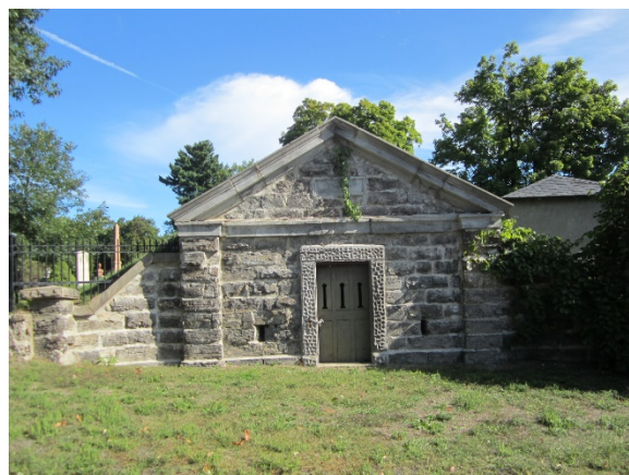
ST. ANDREWS PROTESTANT CEMETERY CHARNEL HOUSE, BUILT IN 1968, IS IN THE FORM OF A VAULT BUILT INTO THE HILLSIDE. MADE OF STONE, IT IS INTEGRATED INTO THE STONE AND WROUGHT IRON FENCE ALONG THE FRONT OF THE CEMETERY (SAA-47-2).
