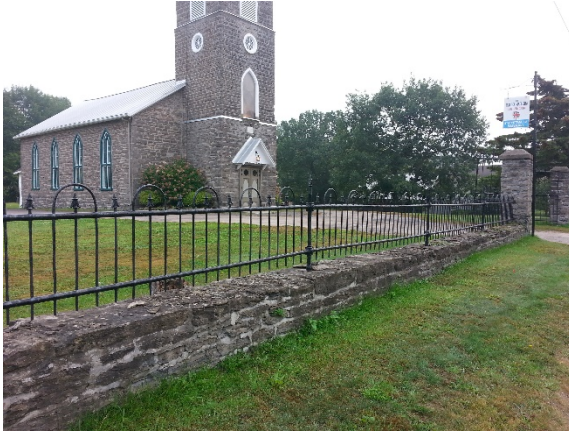
ORNAMENTAL WROUGHT IRON FENCE WITH LOW STONE WALLS AND COLUMNS, ALONG THE FRONT OF ST. MATTHEW' S CEMETERY, GRENVILLE (GREN-18).
