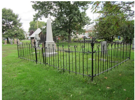
WROUGHT IRON FENCE MARKING THE BOUNDARY OF THE BESWARICK FAMILY PLOT IN ST. MATTHEW'S CEMETERY (GREN-19 FT-4)
